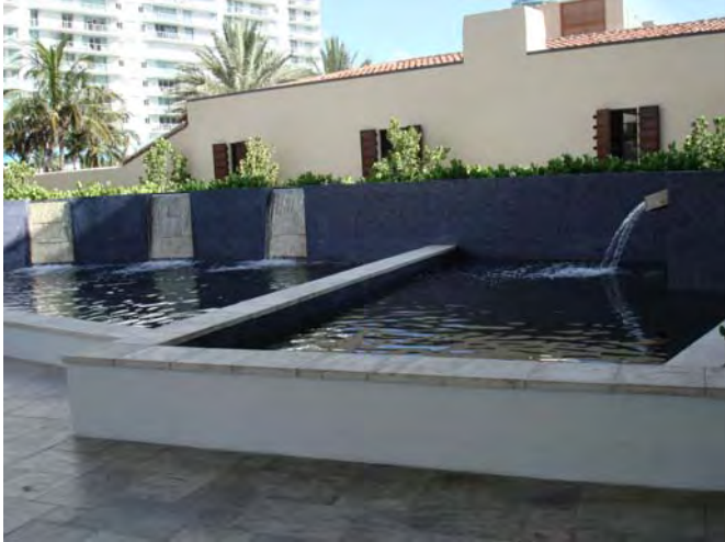
Front Drive Entrance leading to Lobby
