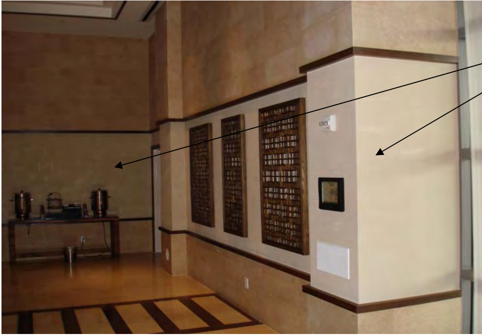
Entering Front Lobby Looking Right
