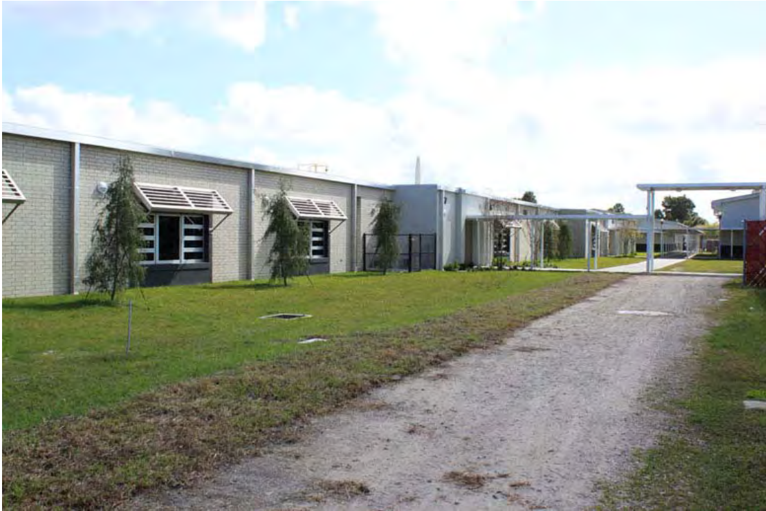
Granyte installed at each window surround
