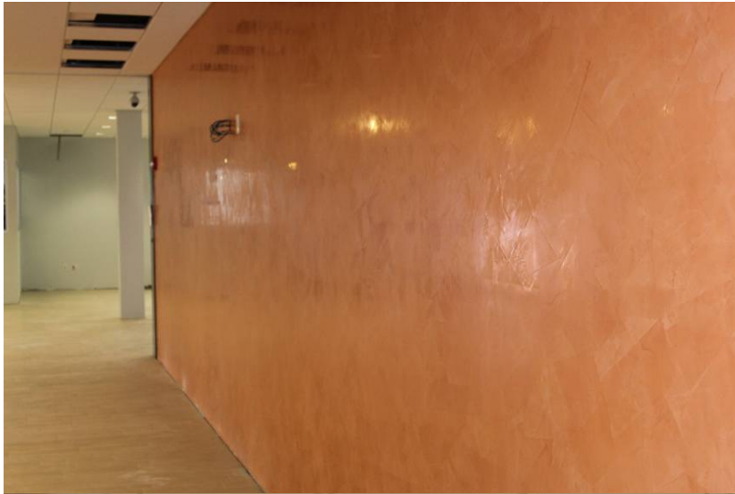
Service Lounge with view towards service bays
