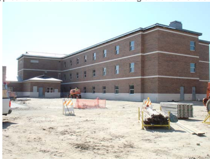
Typical exterior of barracks building under construction
